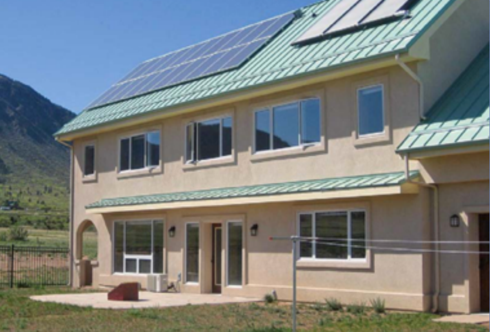
Riggins/Coleman 2011 Monument, CO house. ~100% ambient conditioned, 100% solar water heating, solar clothes drying, net zero electricity. Jim Riggins photo.
