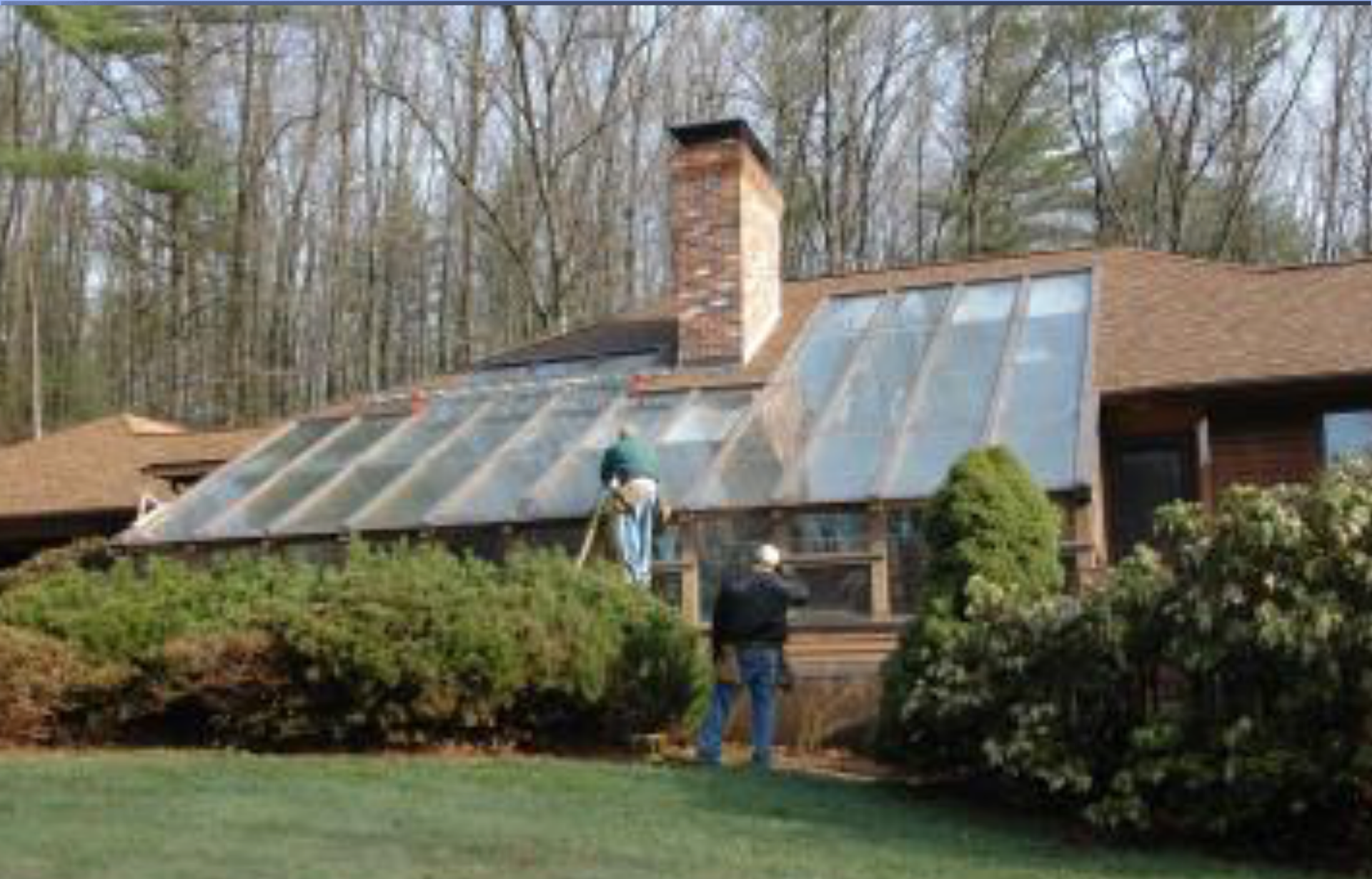
Warren/Saunders Boxborough MA house 1986. (Similar to Saunders Shrewsbury MA house 1981.) R30 walls, 18,000 gal water, 100 tons rock. 65-75 F year-round. WarrenDesign photo.
