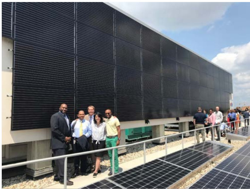
Downtown DC Office Building - 799 9th Street NW, 55kW
