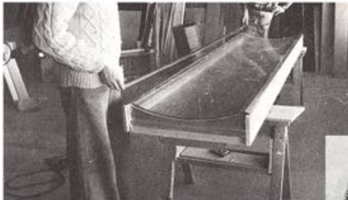
Laying on the glazing caps.
