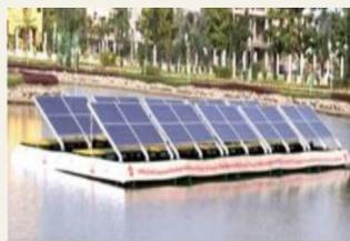
Fig. 1. The Baysh dam near Gizan Fig. 2. A 10 KW FPV plant [7]
