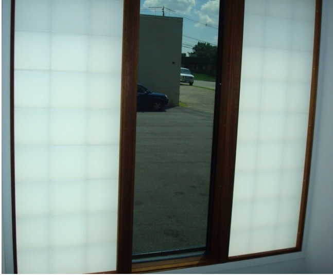
Fig. 8: Solar Window installation used for Colorado test.
