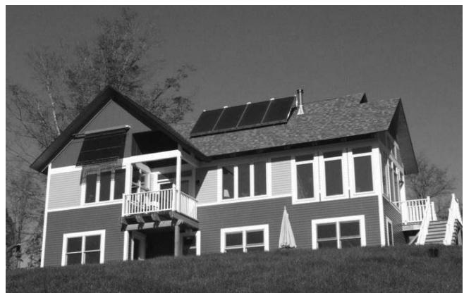
Figure 4: Image of the solar thermal system installed on Home 2. (Source: CARB study)
