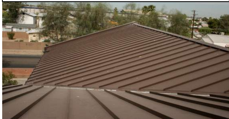
Photograph of the sloped roof area of the Fire Station building.
