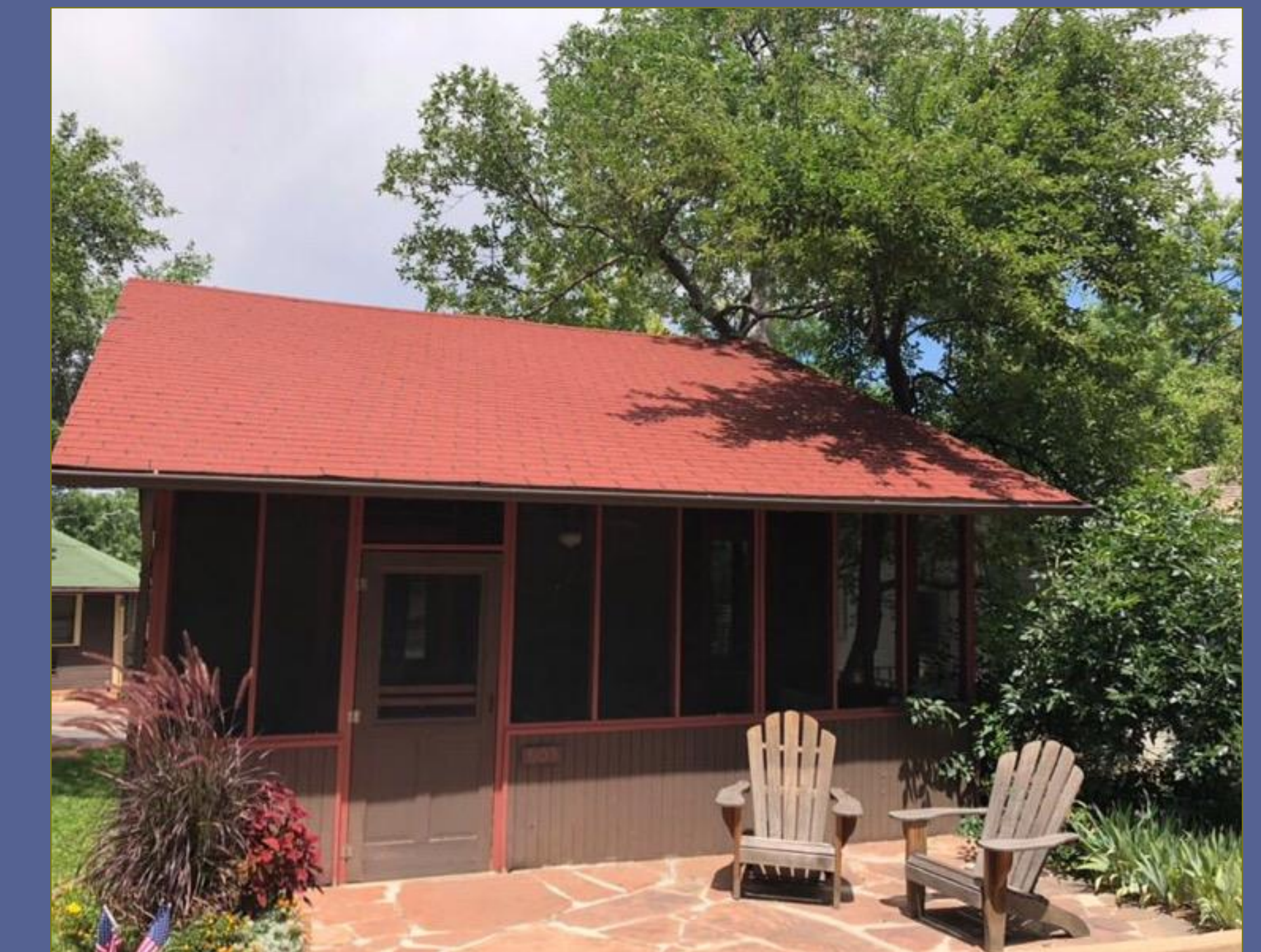
Figure 4. Post installation, there is no visual impact on the primary elevation of the historic cottage.
